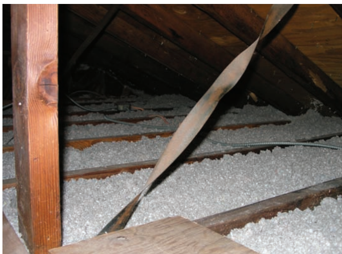
Blown cellulose insulation in attic
