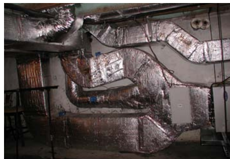
Ductwork sealed and insulated
