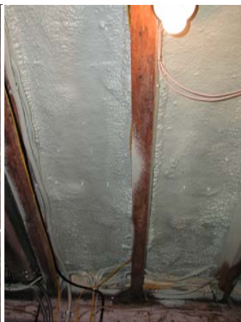
Expandable spray foam insulation*
