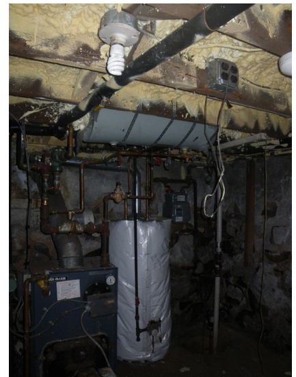
Added insulation in basement (before barrier)*
