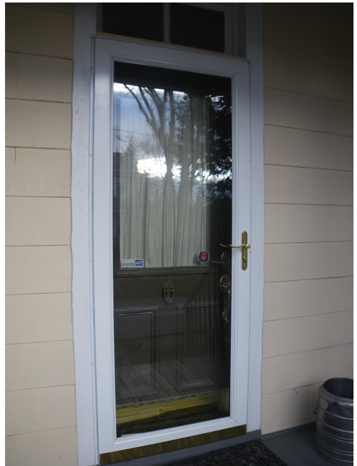
Storm door installed to provide added protection
