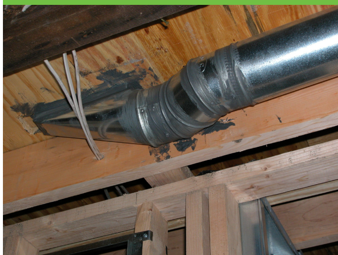
Ducts sealed with mastic
